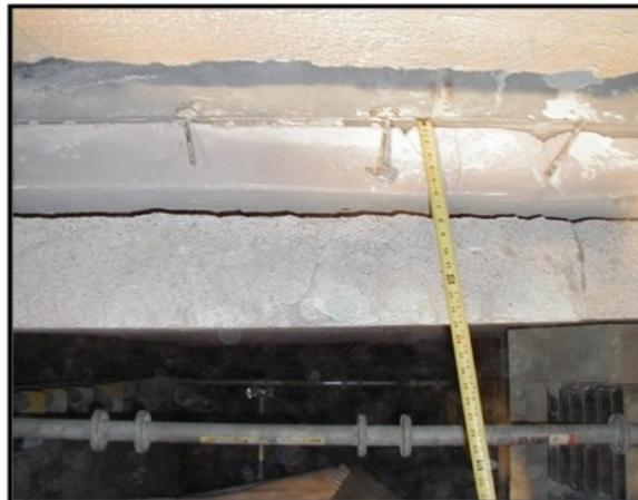
**Figure 1. Example of end result when improper selections are made in anchorage and refractory material for the operating conditions.**
