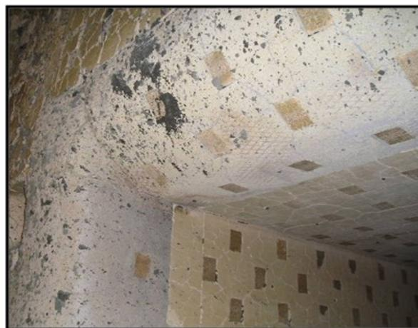
**Figure 2. Improved refractory life utilizing ceramic and wire anchors in cooler hot end bullnose.**
