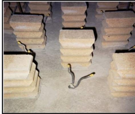
Figure 13. Dual Lining Anchor Configuration Showing Castable Anchored with Ceramic and Wire Anchors and L-Clip.
